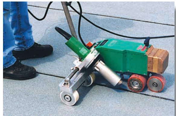
VARIMAT being used to weld modified bitumen membranes.
