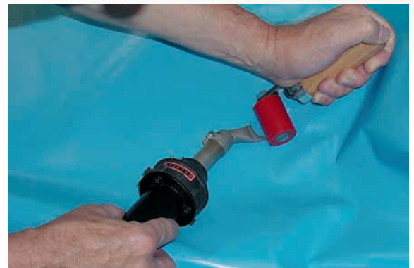
Repairing a pool cover with HOT-JET S.
