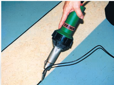
TRIAC S hand-welding tool equipped with speed welding nozzle.
